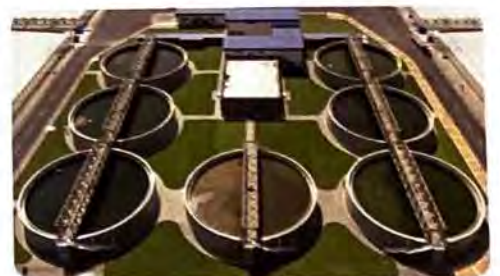
Bahr Al-Baqar wastewater treatment plant
